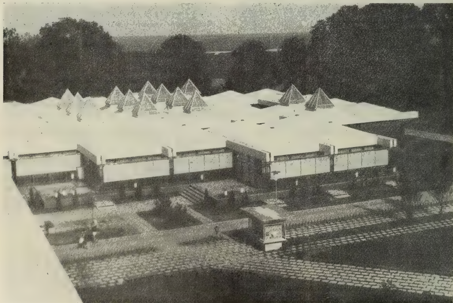
The prefabricated bungalows are illustrative of the builders' rich fantasy
